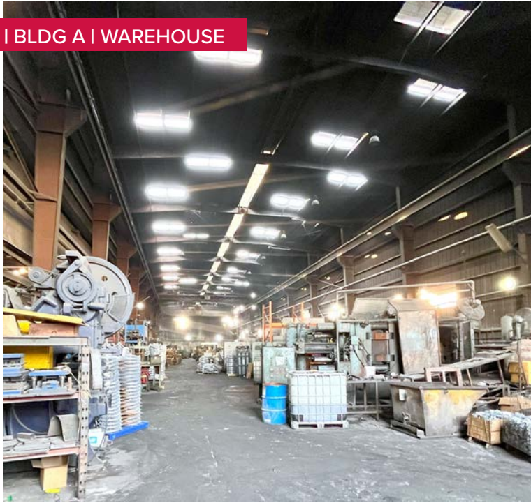
I BLDG A | WAREHOUSE CRANES
