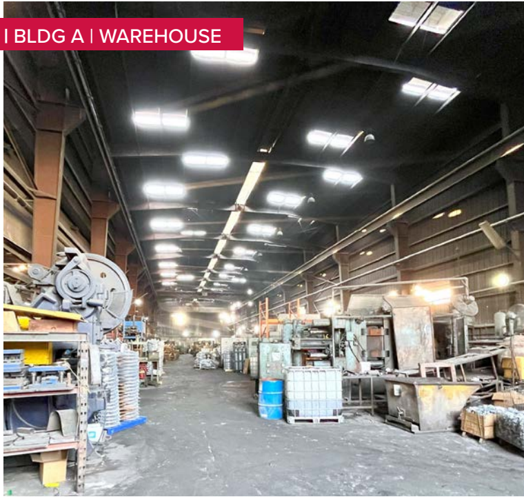
I BLDG A | WAREHOUSE CRANES
